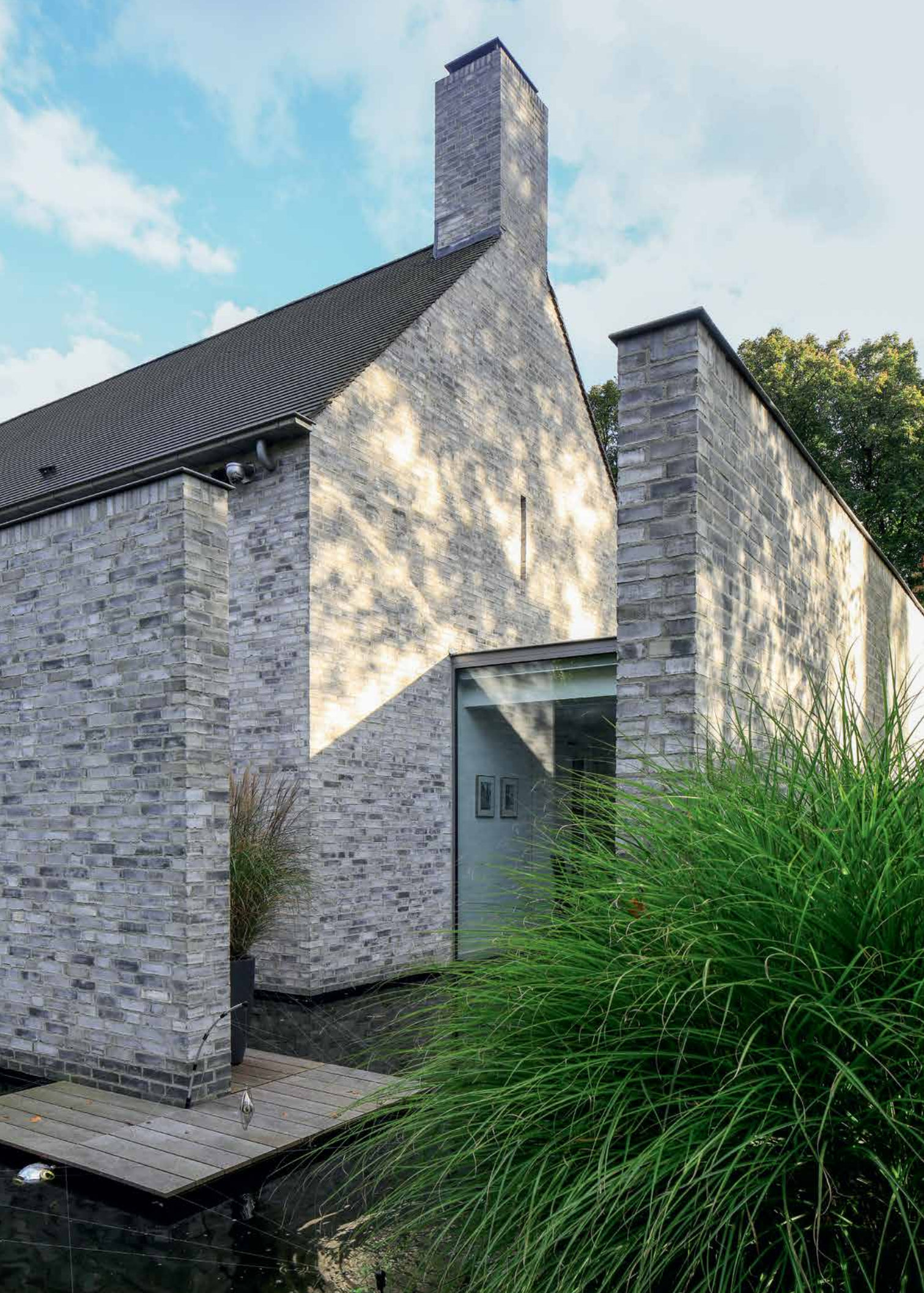
Villa Rotonda is tight and precise, with gable-end chimneys and a 44-degree pitched roof.
