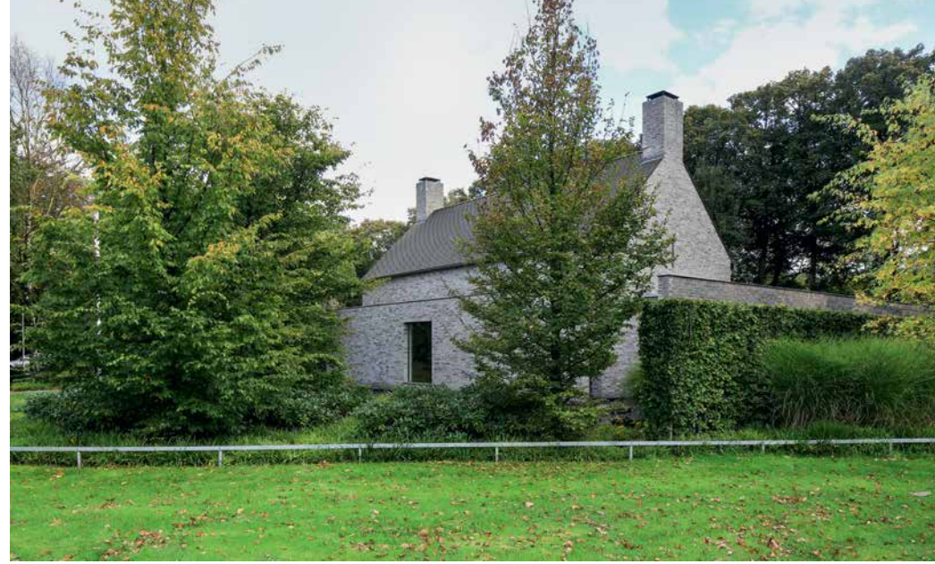
The building is on a corner, and is flanked by two roads and a roundabout, from which it shields itself off.
